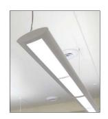
The upgrade included retrofitting the existing two row continuous runs made of twelve four-foot 2-F32T8 fluorescent fixtures with two rows of Metalumen's six eight-foot continuous runs using Orbit O2DS LED luminaires (35W/four-foot). As a result, our electrical load was reduced by 55% in the Education Centre, resulting in a projected annual energy savings of \$442 (1,880 kWh) with a **0.59-year payback**.
